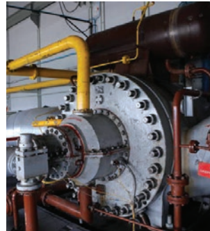
Equipment condition & reusability
