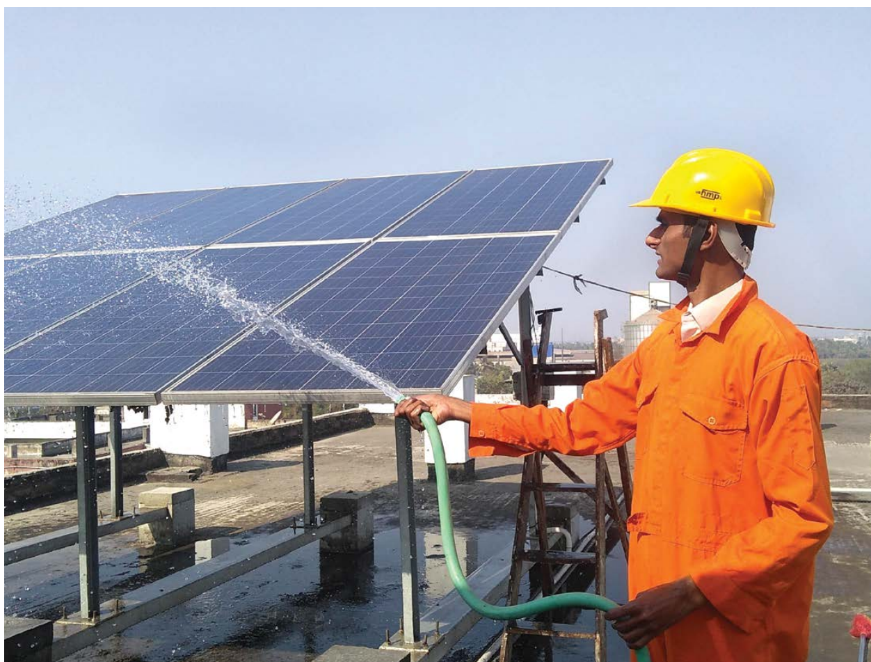
A worker cleaning a solar panel/ Arpo Mukherjee, iFOREST
