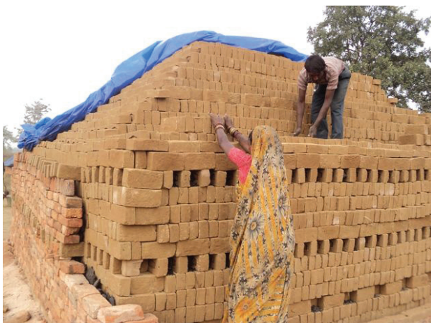
Arrangement of bricks in a clamp
