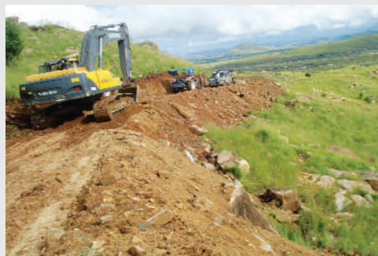
Vegetation destroyed on contours and other parts for road construction for windmill material transportation
